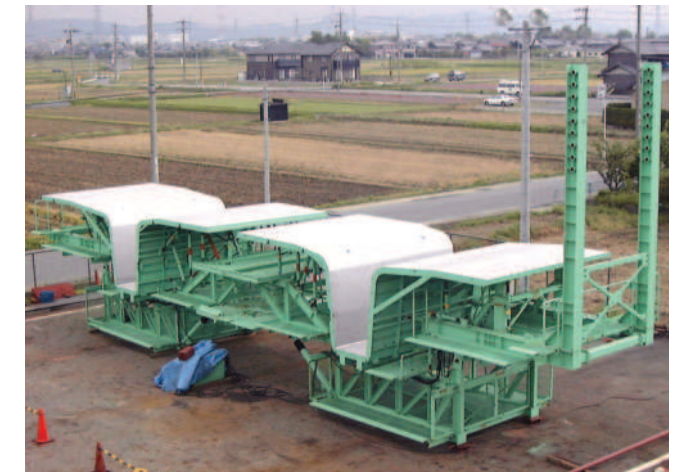
MOVING STEEL RIG MADE OF READY-MADE STEEL PLATE
