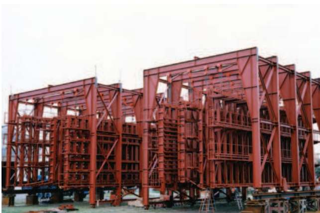
沈埋函型枠 IMMERSED TUBE SLIDING FORM
