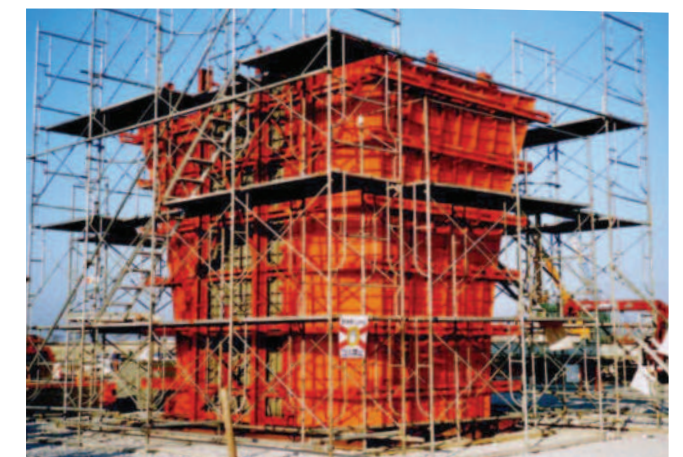
3次元橋脚型枠 THREE-DIMENSIONAL PIER FORM
