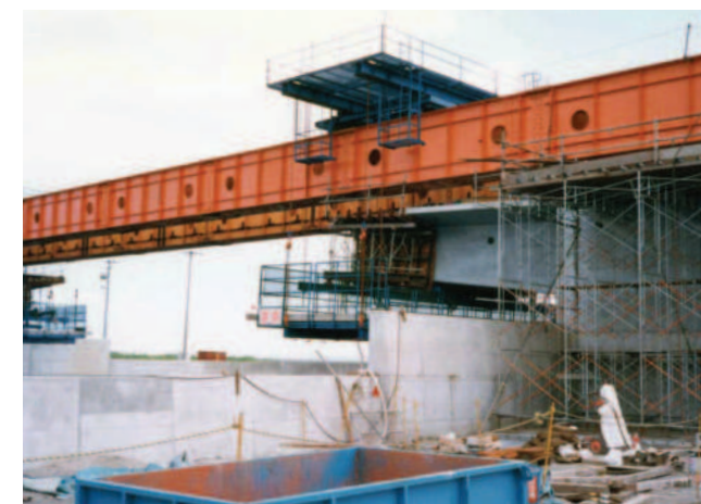
架設移動台車 CONCRETE SLAB LINING LIG
