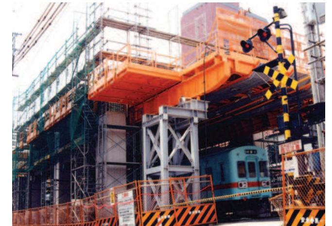
直上高架橋移動支保工 MOVING STEEL RIG FOR OVERHEAD BRIDGE
