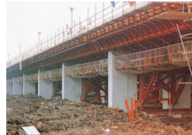
架設移動台車 CONCRETE SLAB LINING LIG
