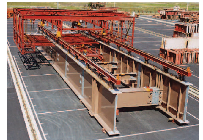
直上高架橋移動支保工 MOVING STEEL RIG FOR OVERHEAD BRIDGE
