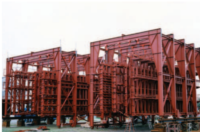
沈埋函型枠 IMMERSED TUBE SLIDING FORM
