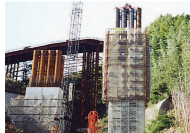
ピア型枠施工用移動足場 MOVING SCAFFOLD FOR PIER FORM CONSTRUCTION
