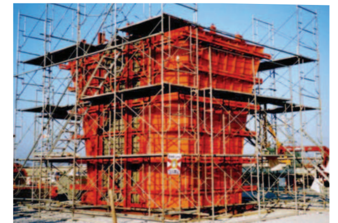
3次元橋脚型枠 THREE-DIMENSIONAL PIER FORM
