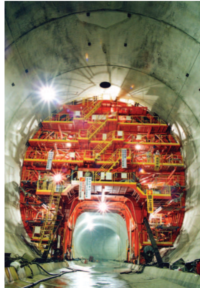
変断面SS SLIDING FORM FOR VARIANT SECTIONS
